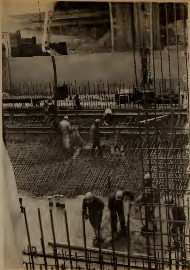
Pouring of concrete for invert by a pumper.
